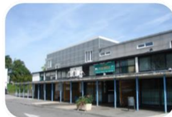
Construction salle de sport associative
